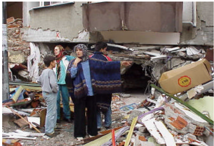
A group of Turkish citizens look over the damage caused by the earthquake in the city of Izmit, southeast of Istanbul
