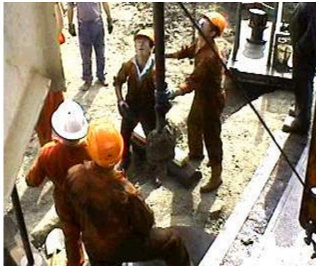
Tempest Environmental Systems drills wells at Camp Hope
